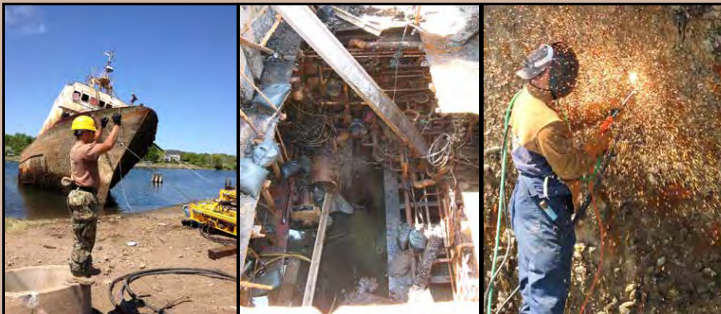
Left to Right: Navy Diver Chief Jason Gray directs hydraulic puller operations during the beaching of Cape Ann III in Sydney, NS on 27 May 2012; A view of the engineroom on Cape Ann III where Navy Divers spent four days installing patches; Navy Diver Second Class Martin Horan cuts an access hole in the bow of Cape Ann III so that three sets of chain can be rigged to the ship to support the final beaching pull.
