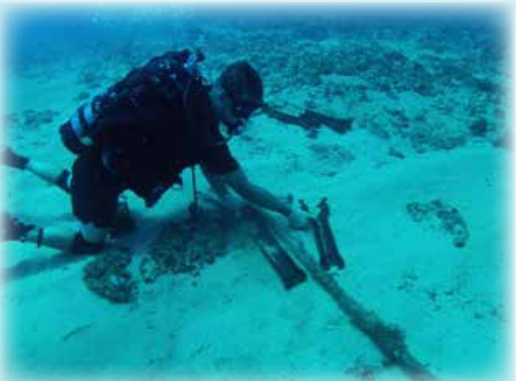
CEC (SCW/MDV) Terry Juergens installing split pipe on cable, PMRF Kauai, HI.
