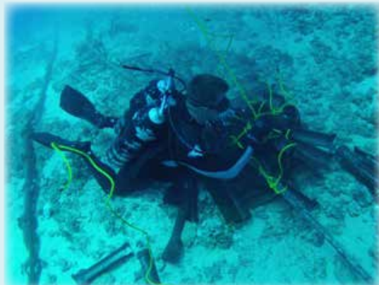
SW2 Oswald preparing split pipe for installation, PMRF Kauai, HI.
