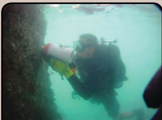
CM1 (SCW/DV) James Richardson conducting ultrasonic thickness measurements to establish remaining thickness of steel caissons.
