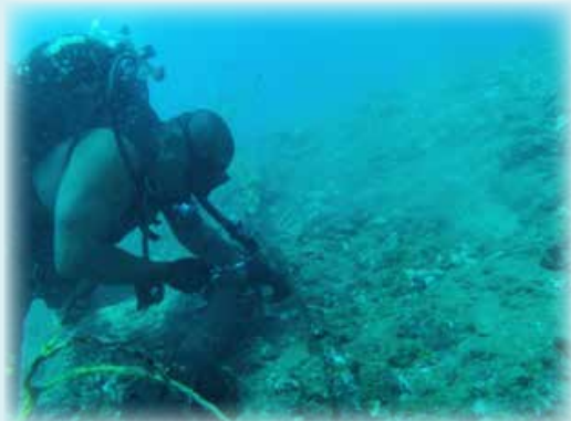
BU1 Wedekind installing bolts on split pipe, PMRF Kauai, HI.
