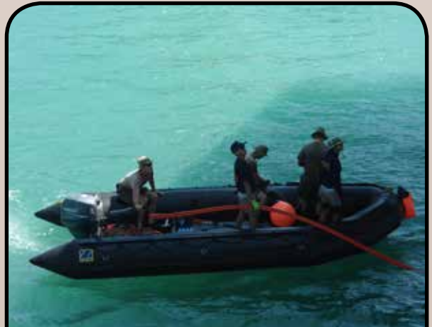
UCT-TWO and Royal Thailand Navy Seabee Divers setting up for hydraulic drilling operations on Throng Prong Pier.
