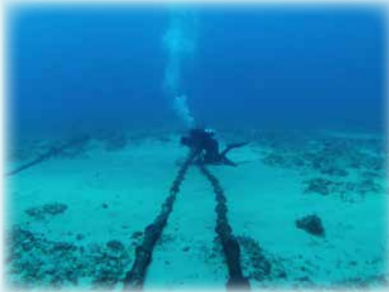
SW1 Sligo installing cable tags, PMRF Kauai, HI.
