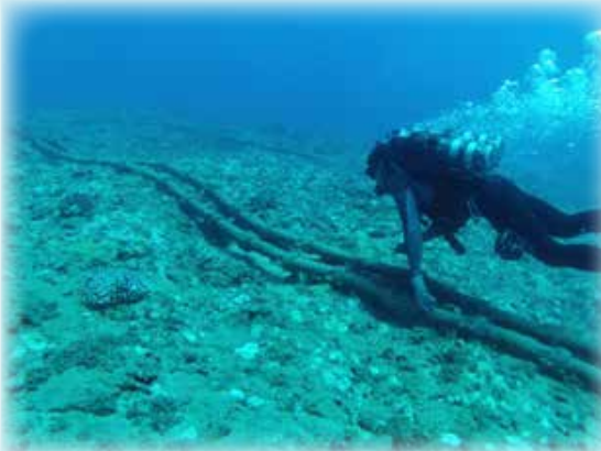
SW1 Sligo inspecting installed split pipe, PMRF Kauai, HI.
